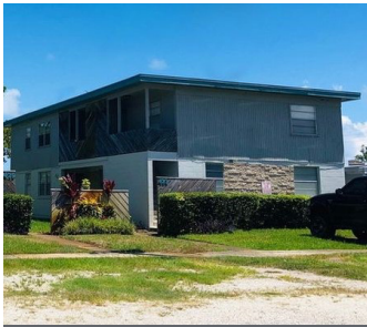
429 9TH AVENUE NORTH 4 UNITS | BEACHES
