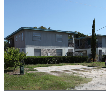
423 9TH AVENUE NORTH 4 UNITS | BEACHES
