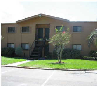
LANDINGS AT PARK VIEW 68 UNITS | SOUTHSIDE
