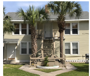
217 12TH AVENUE NORTH 2 UNITS | BEACHES
