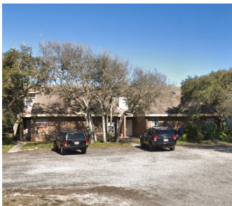
SEAGATE APARTMENTS 4 UNITS | ST. AUGUSTINE
