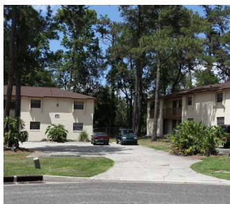
SEABOARD OAKS 76 UNITS | WESTSIDE
