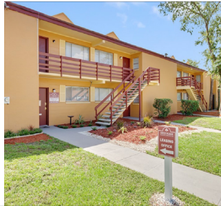
ARCO PLACE APARTMENTS 48 UNITS | ARLINGTON
