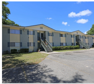
LINDA APARTMENTS 48 UNITS | CENTRAL JAX
